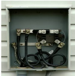
Step 2a Hi-Lug Ground Installation
