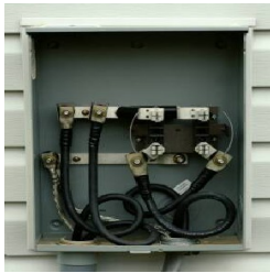
Step 2a Hi-Lug Ground Installation
