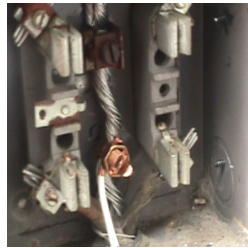
Step 2b Split-nut Ground Installation
